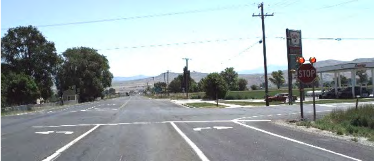
Figure 13: Old Configuration with Flashing Red Lights Mounted Above Stop Signs
