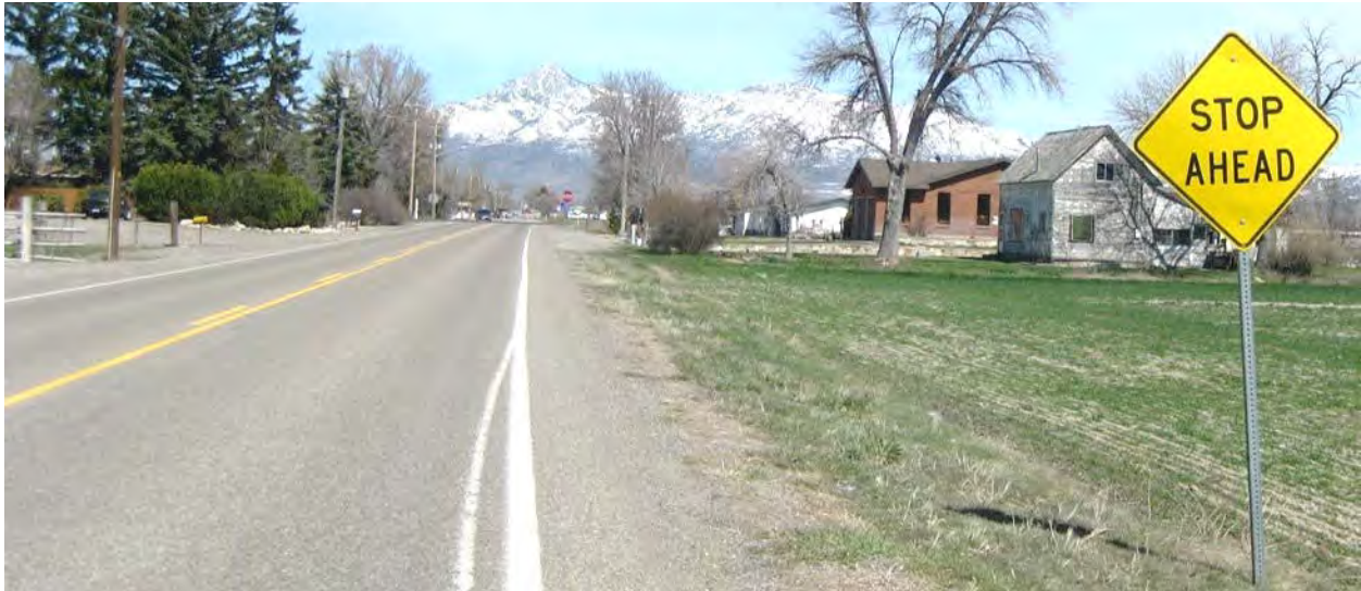
Figure 16: Northbound Approach Advance Warning Features
