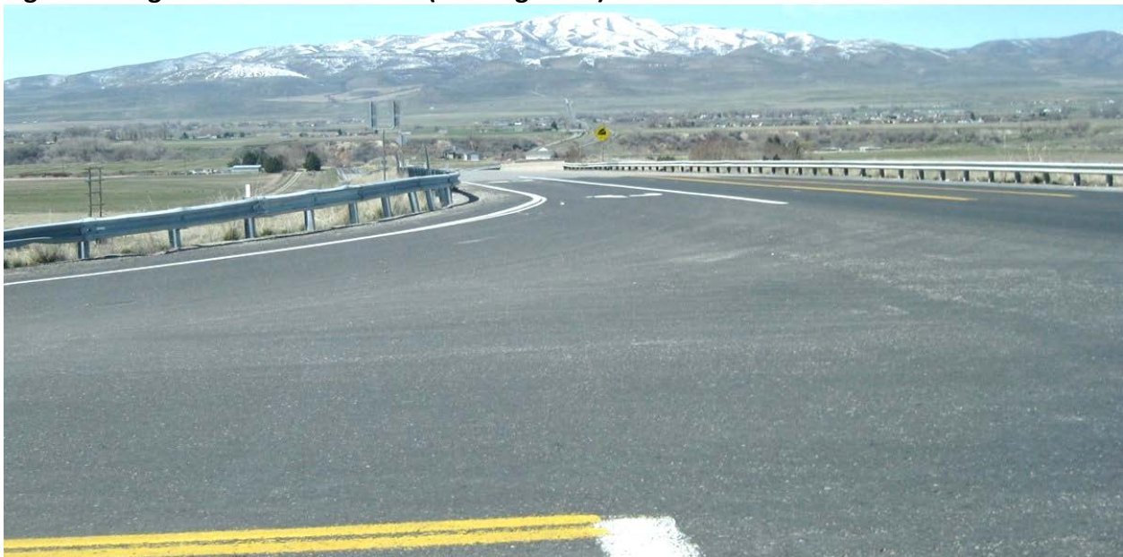
Figure 20: Sight Distance on S.R. 38 (Looking West)
