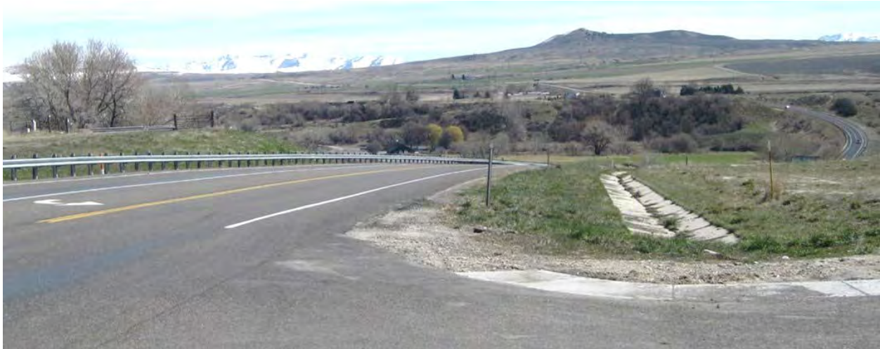
Figure 24: Sight Distance at Bear Hollow Drive (Looking East)
