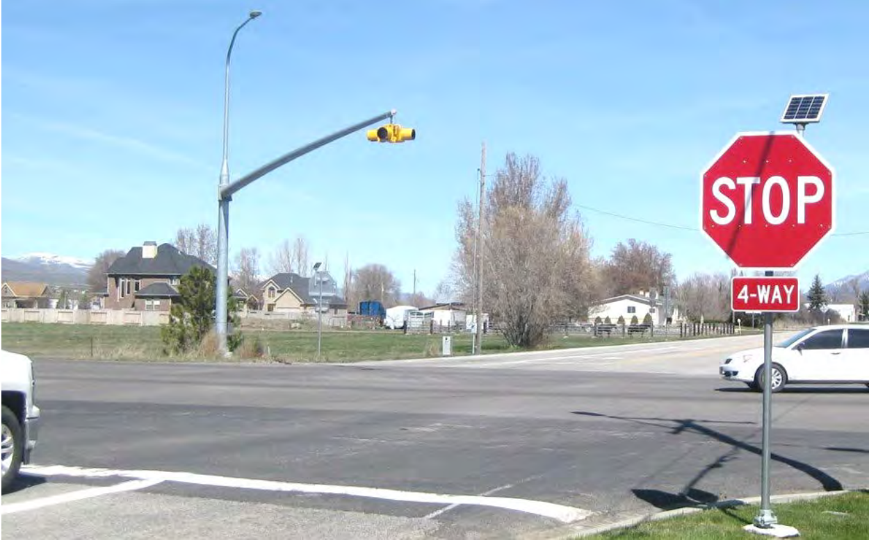
Figure 14: New Stop Signs and Overhead Flashing Red Above Center of Intersection
