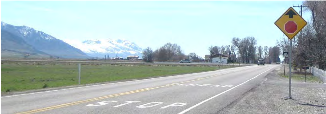
Figure 17: Southbound Approach Advance Warning Features
